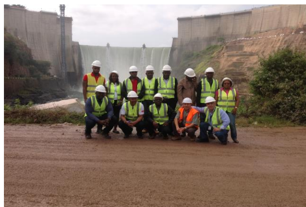
PDRI Team pose for a photo during a site visit at Campambe I and II Dam wall that is being raised to achieve the required head
