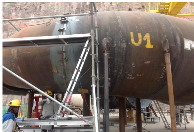
Construction works in progress at Campambe II power station
